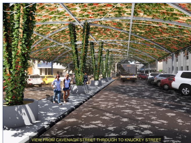
Figure 2: The 50-metre canopy structure is designed to reduce ambient temperatures in the CBD, NT Government
